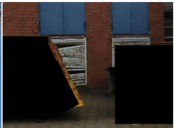
Lamellengitter schadhaft
